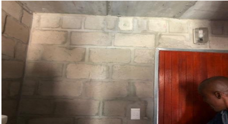
Figure 4.6: Un-plastered internal walls in Joe Slovo houses
