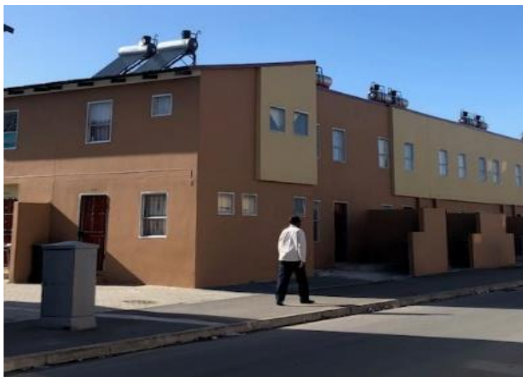
Figure 4.3 Slovo Park Phase 3 - SWH installation
