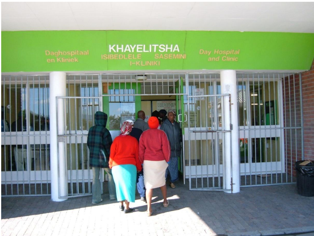
Figure 9: Entrance to the Site B day hospital
