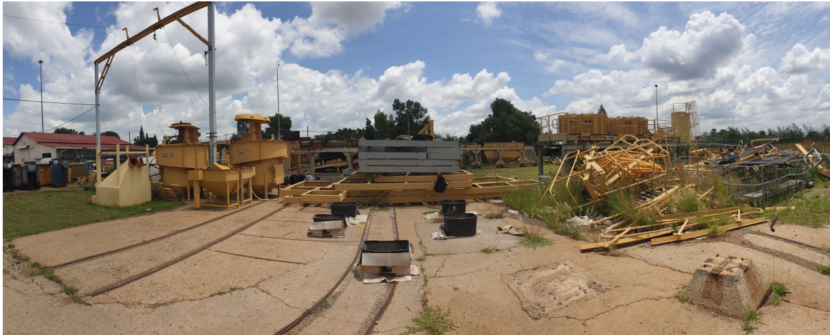
Figure 4.2: Mining company workshop, cnr Bridges ave and Cedar lane, Westonaria, 1781
