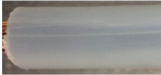
Figure 3.3: XLPE Tram Line Defect
