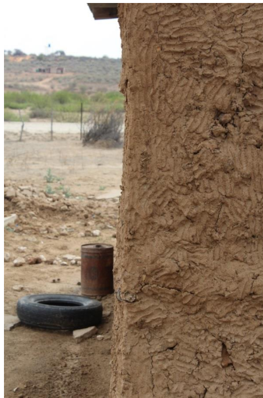
Figure 89 Finger indents from the process of making. Author (2015)
