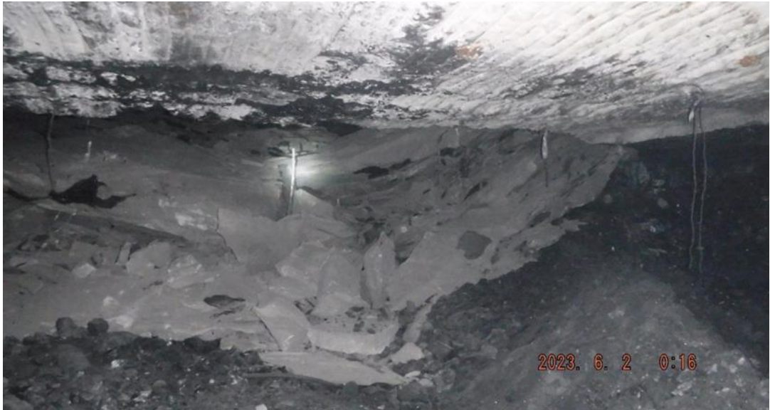
Figure 1-2: Failure of the roof in a New Denmark Colliery pillar extraction section, known as goafing.
