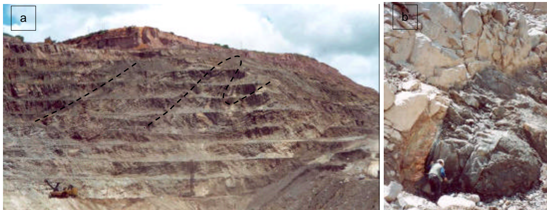
Figure 4.16. (a) The isoclinally folded Dolomite Schist in the hangingwall of the Upper Orebody in the Nchanga open pit is resultant of compressional deformation during Lufilian orogenesis. (b) A phlogopite-scapolite schistose unit in the Nchanga open pit has been described by various authors as a lamprophyre dyke (Diederix, 1977), a metamorphosed gabbro (Fleischer et al., 1976) and as fault gouge (McGowan, 2003).
