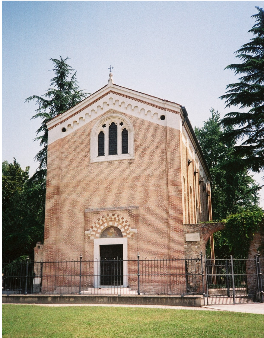
13. Exterior of the Arena or Scrovegni Chapel, Padua, Italy, 2004. © Jeannine Howse.
