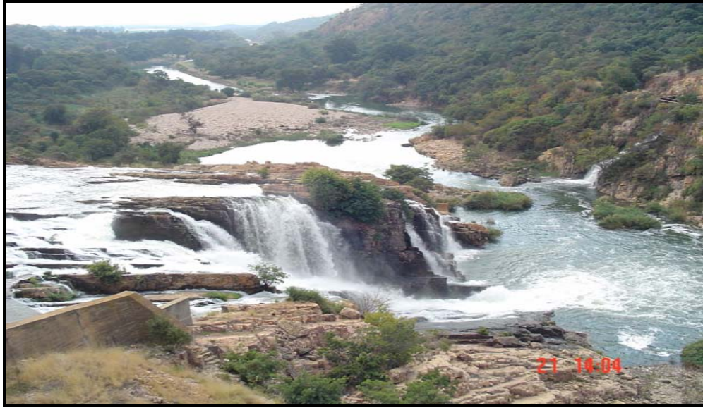
Figure 2.7: Natural aeration as observed in Crocodile River about 50 m downstream the outflow of the Hartbeespoort Dam.
