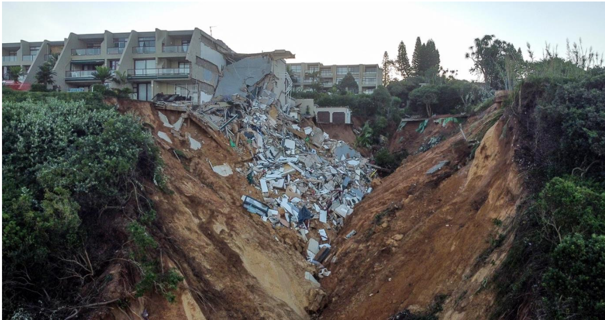
Figure 2.2: 2022 landslide damage in KZN after floods (MacRobert, 2022).
