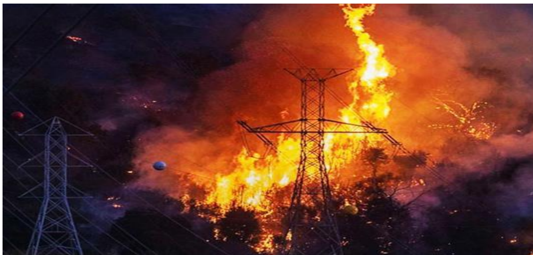
Figure 5: Intense lightning impact on electricity infrastructure (Insulator News and Market Report, 2021).
