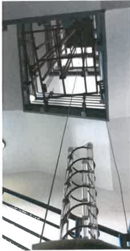
Figure 6.20 Test Antenna in CoM Vertical Shaft
