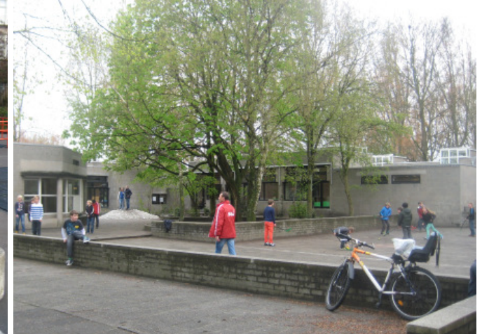
figure 119: Hertzberger. Montessori School . Delft, 1944-1947 (site visit, 2012).
