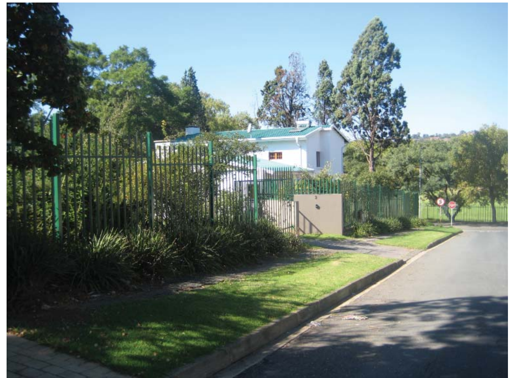
figure 66d: The remaining residential house on the site. Located corner Avonwold Road and Newport Road.
