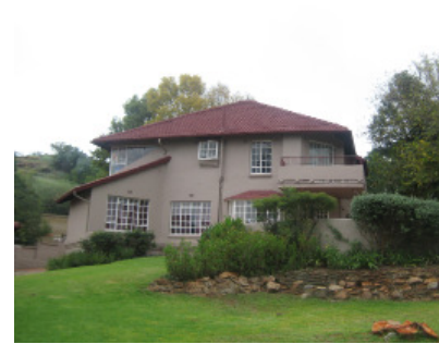
figure 9b: Post-80s Johannesburg Children's Home.
