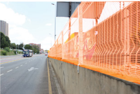
Fence between a raised sidewalk and Empire road.
