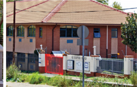
Direct pedestrian entrance to an office park.
