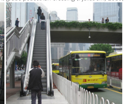
Figure 3m: Escalators connecting the sidewalk with the footbridge (Fjellstrom, 2010)
