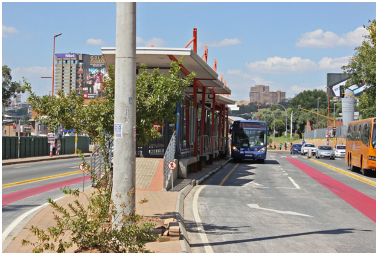
Figure 1a: Object of Research: Rea Vaya – BRT station and bus (Author, 2017).
