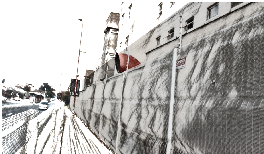
Figure 4p: UJ Sophiatown Student residence clear-vu fence and internal hard wall.
