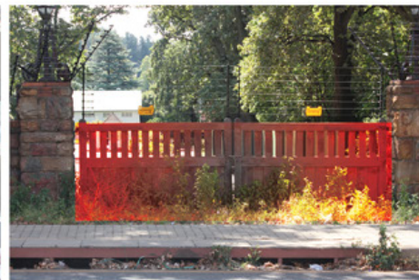
Unused entrance to private property.
