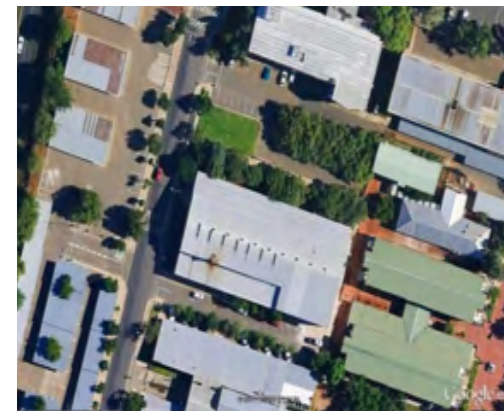
Figure 85: Aerial view of the school building before extensive renovations (centre), UC (Google Earth)
