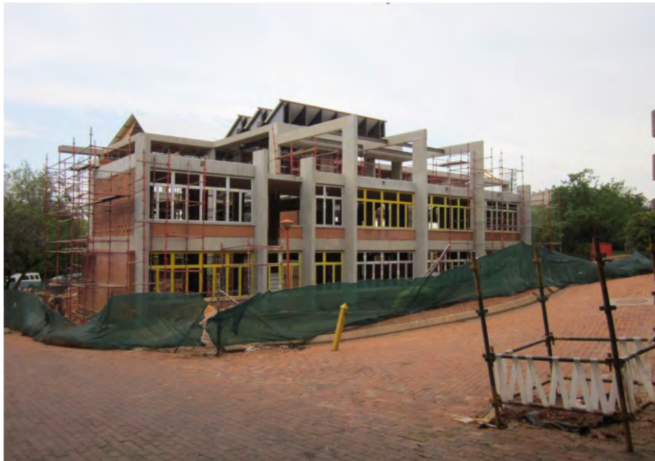
Figure 101: New building for school of architecture under construction, UD (Author, 19.09.2011)
