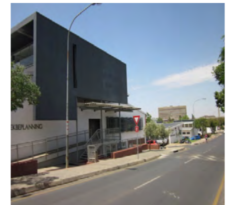
Figure 86: Street / west elevation of the renovated school building, UC (Author, 17.11.2011)
