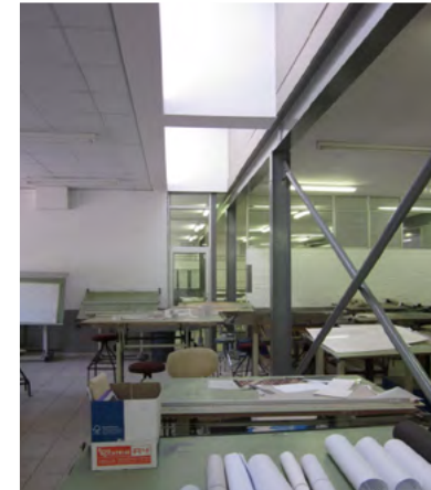
Figure 89: Natural lighting and air ventilation via light wells in large studios (Author, 17.11.2011)
