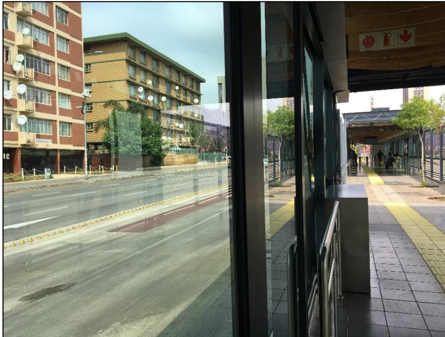
Figure 10: BRT station glass façade
