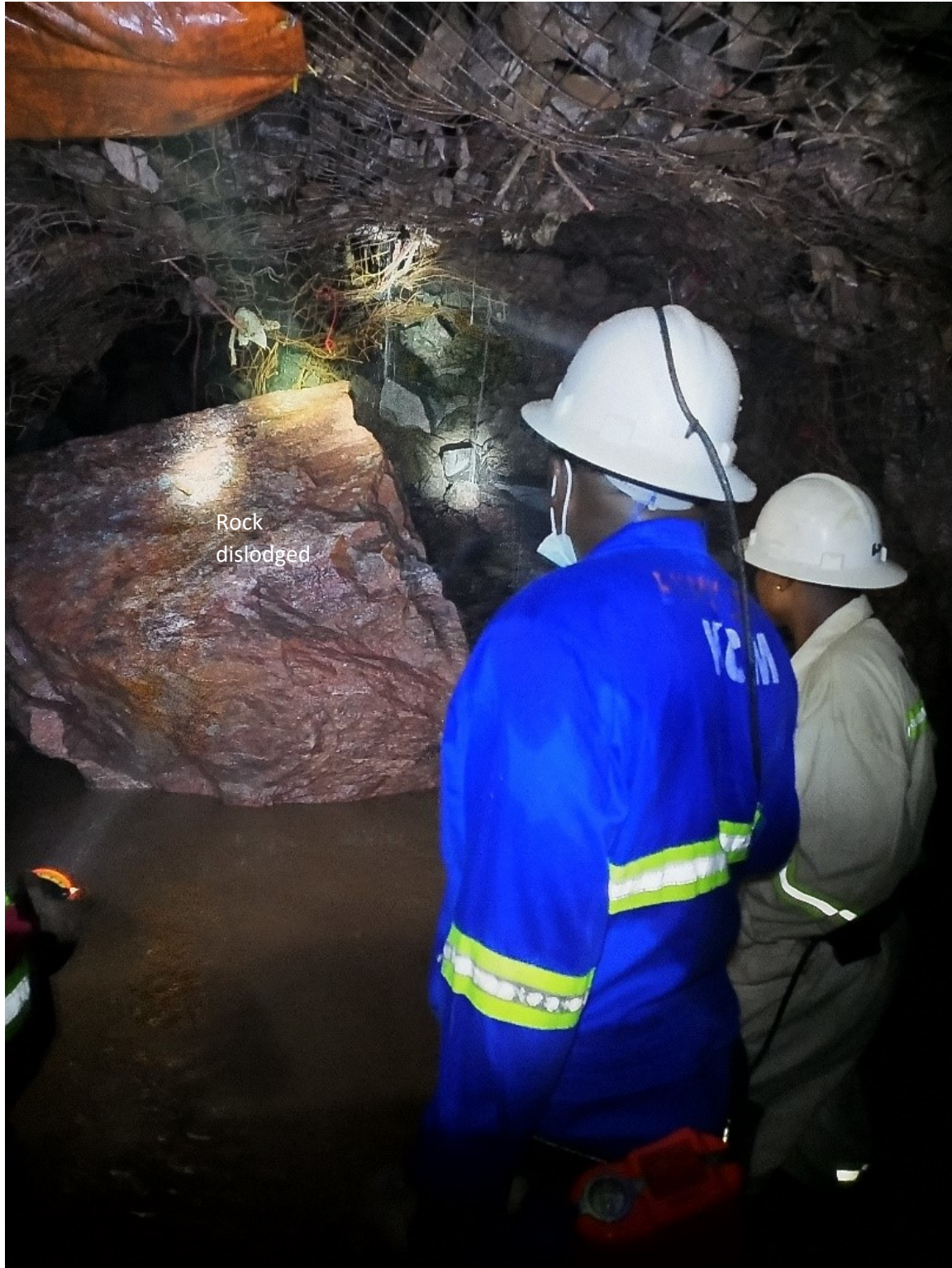
Figure 8-3: Picture of rock dislodged due to wedge failure on 760mL 2400mW access to the ore body.
