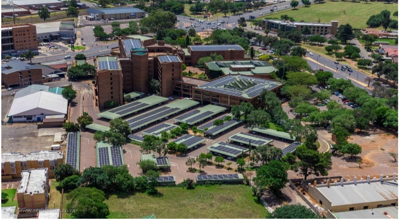
Figure 5.8: Aerial view of the Kempton Park Civic Centre showing the installed rooftop PV system.25 February 2018.
