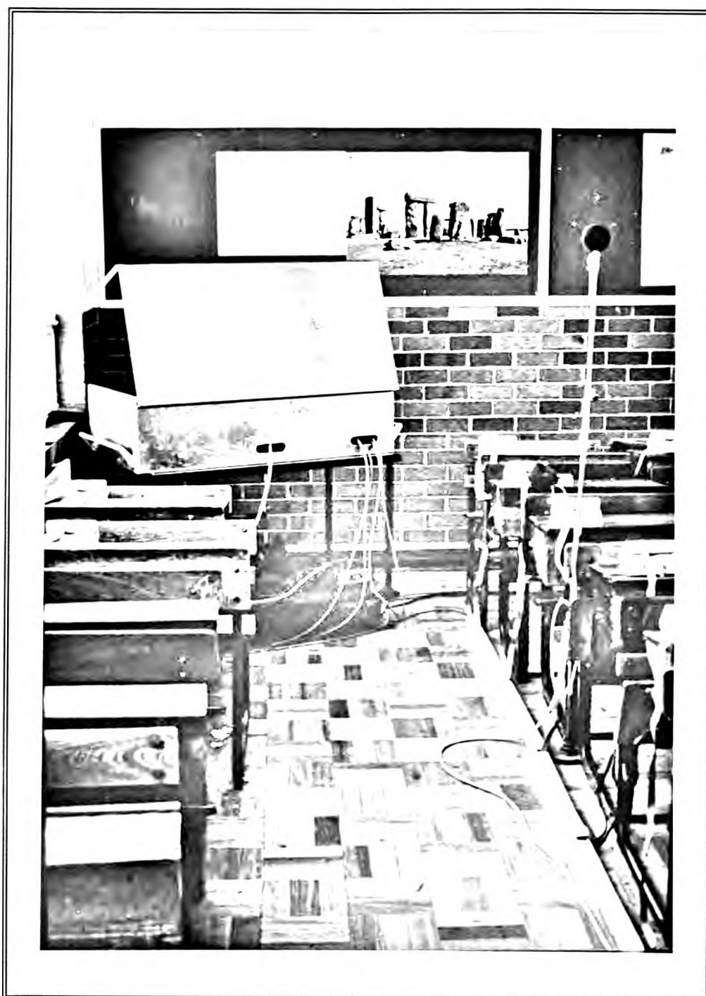
Figure 2.2-11: ADCS control system and cable connections in a classroom.
