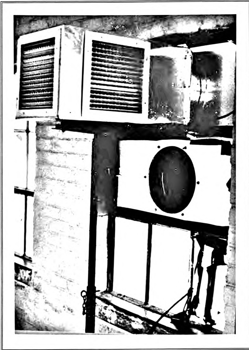
Figure 2.3-3: Air distribution box for temperature control in classroom.
