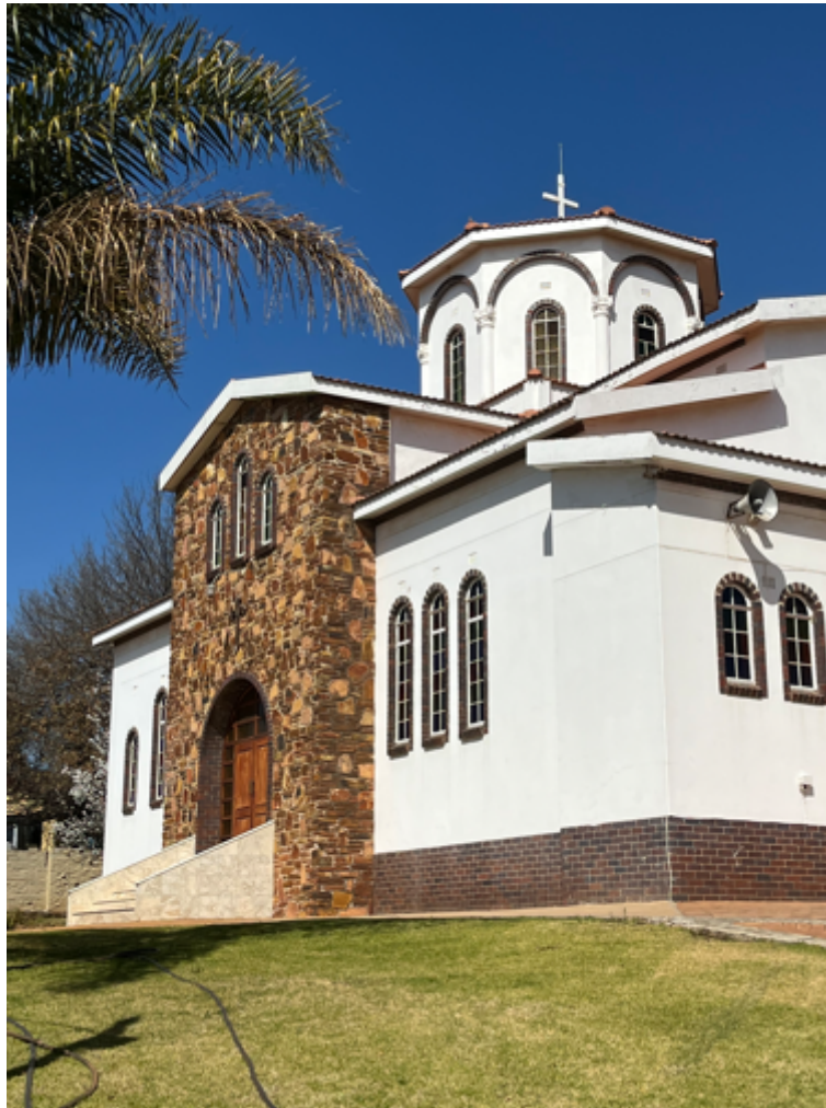
Figure 67: St Andrew's Greek Orthodox Church in Krugersdorp, western Johannesburg
