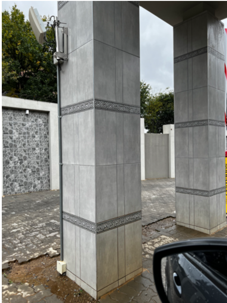
Figure 38: Pillars with a meander pattern at the entrance to the Greek Sporting Club
