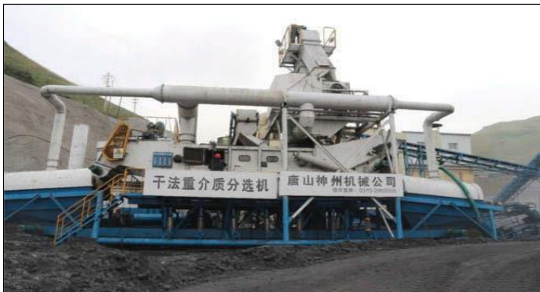
Figure 2-2: World's first modularized dry coal beneficiation plant (Source: Zhao et al. , 2016)
