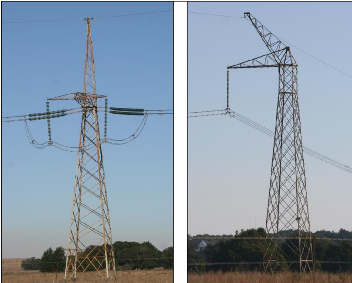
Figure 9: Mono-polar strain and suspension pylons of the Cahora-Bassa HVDC scheme 6 .
