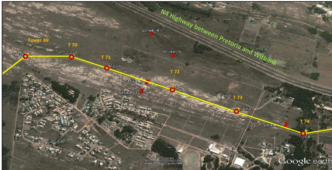
Figure 81: Aerial view of the affected Line 1 section between towers 69 and 74 45 .
