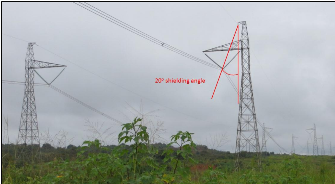
Figure 15: Mono-polar structures of the Inga-Kolwezi HVDC scheme 11 .
