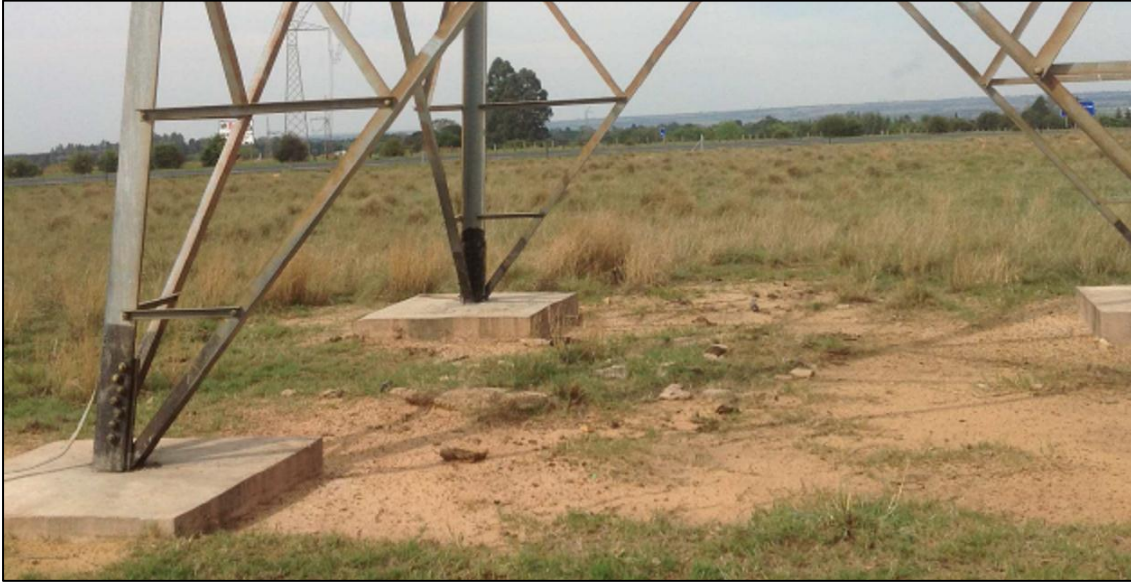
Figure 86: Soil conditions near tower 77 (Miya, 2014b).
