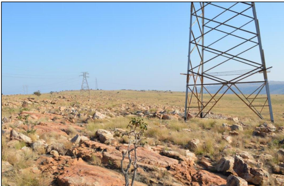
Figure 83: Typical local geological conditions near towers 69 – 74 (Pretorius 2014a).
