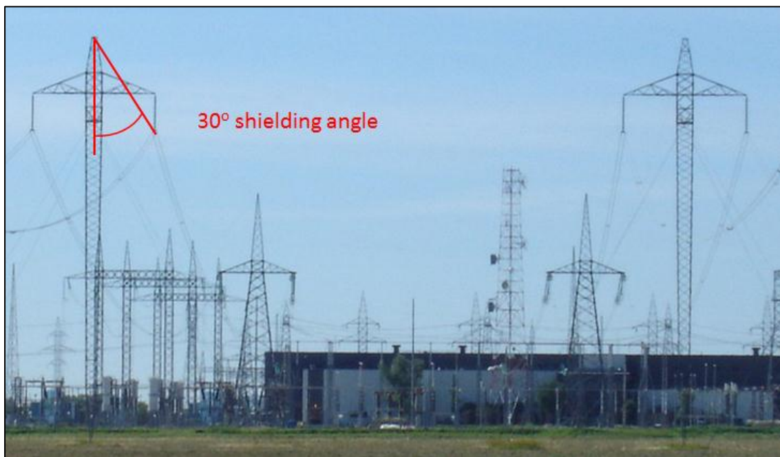
Figure 17: Structures for the Nelson River number 1 and 2 bipoles at Dorsey CS 13 .
