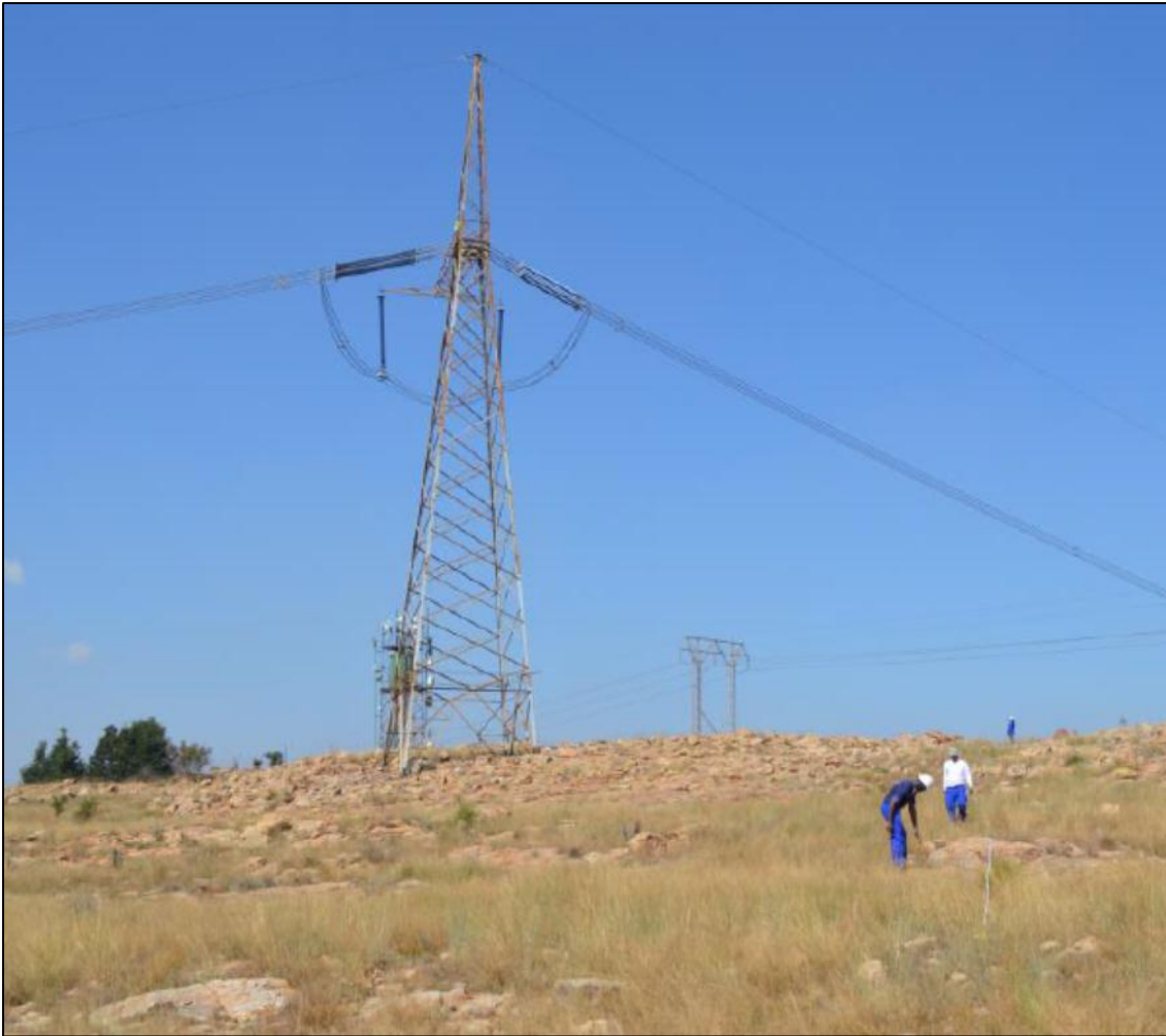
Figure 88: The elevated position of tower 69 (Pretorius 2014a).
