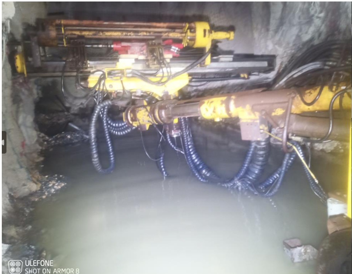
Figure 4-26: Water-logged drilling face, no pumping occurring
