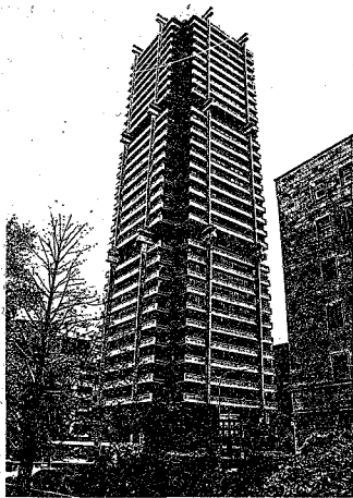
Figure 3: HENTRICH BERGS & ASSOCIATES. Standard Bank Centre. Johannesburg, 1970.
