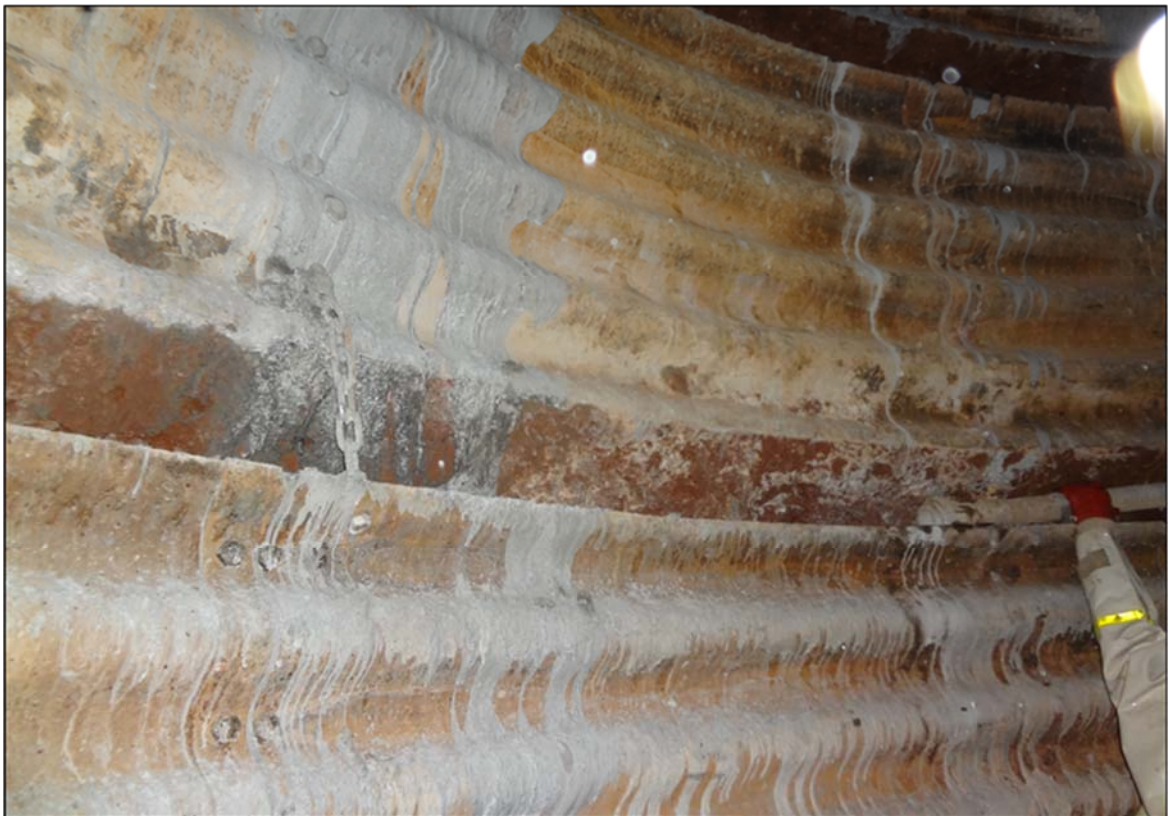
Figure 27: Use of ARMCO back shutters as temporary support in the red clay
