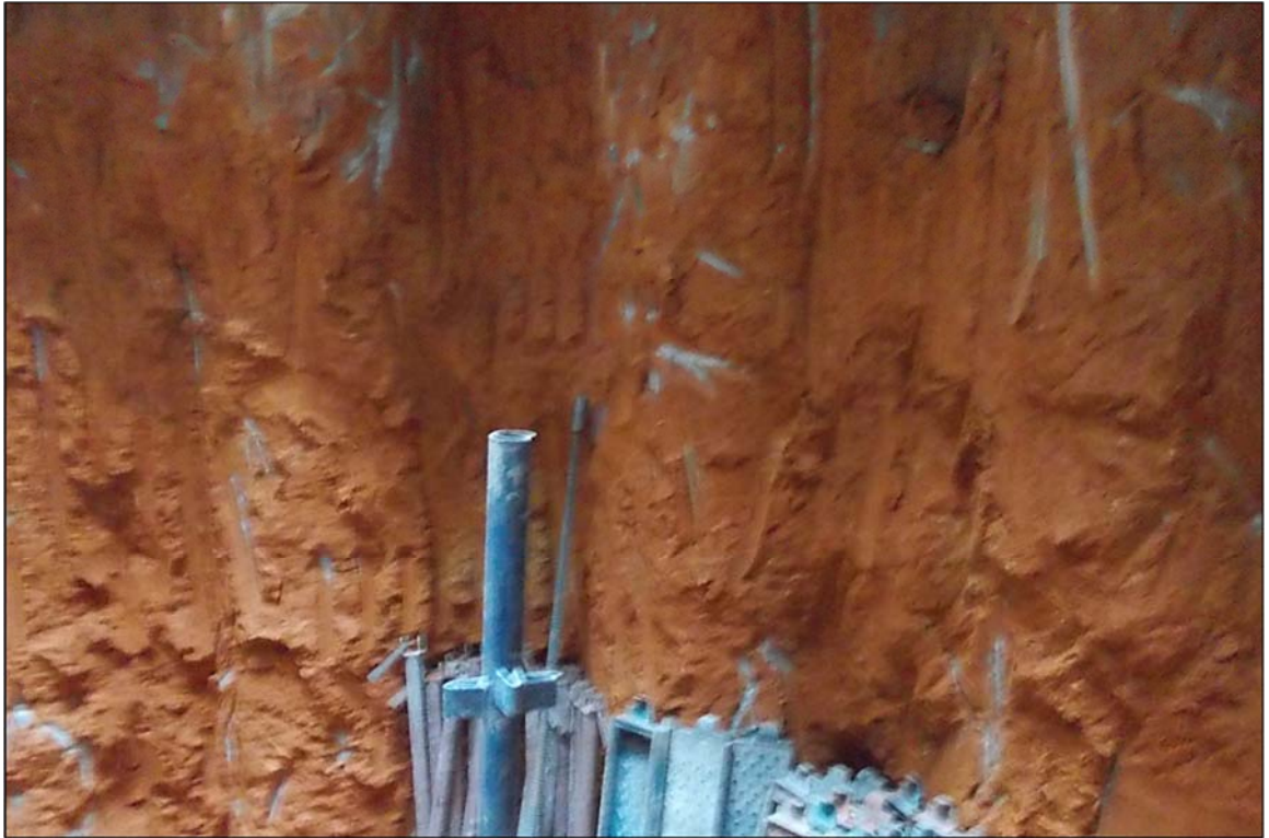
Figure 26: Use of oscillator piles as temporary support in the sands
