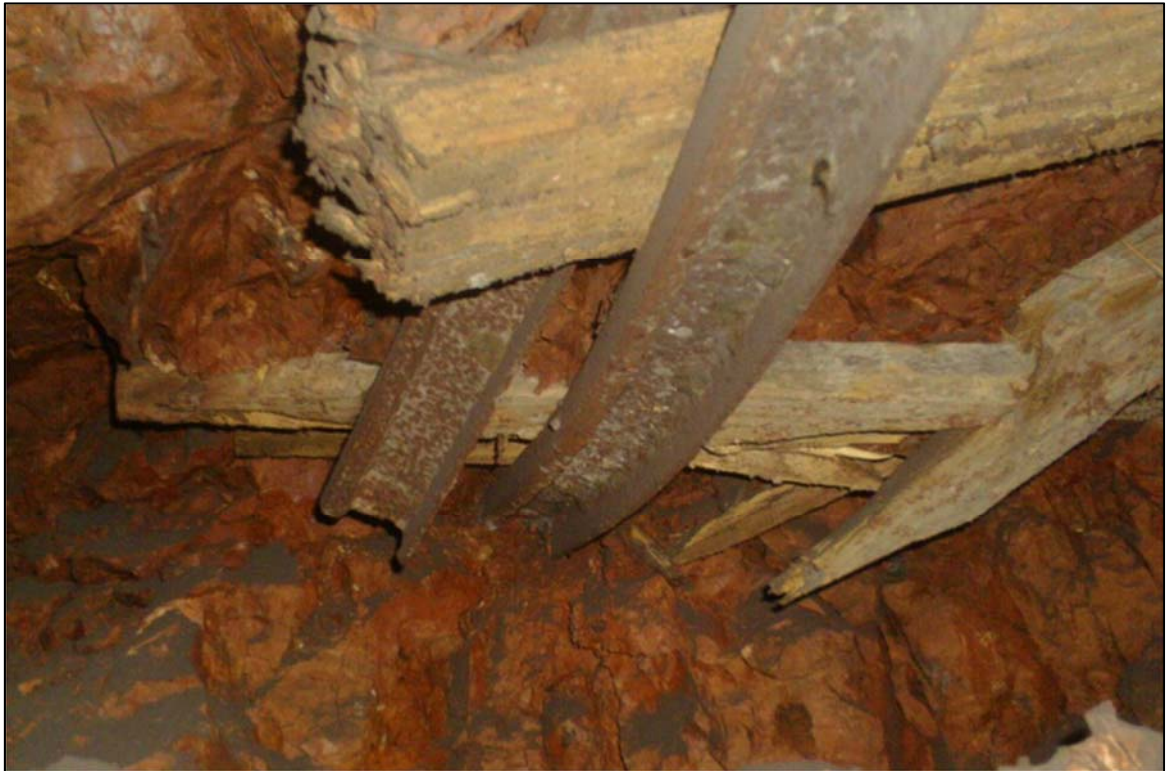
Figure 35: View inside a void showing cribbing support along the red clay section of the decline.
