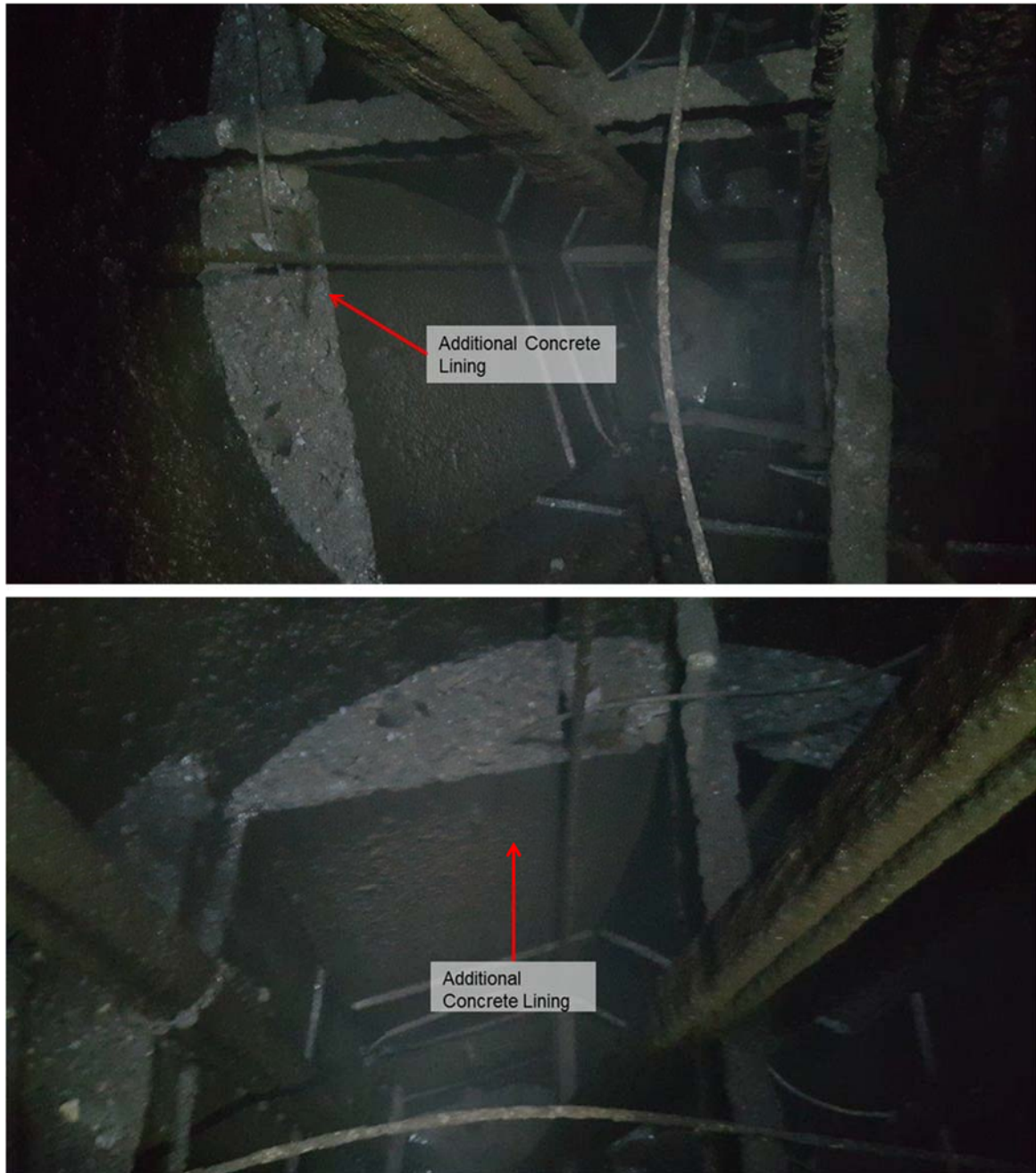
Figure 37: Additional Lining Installed in Red Clay Horizon
