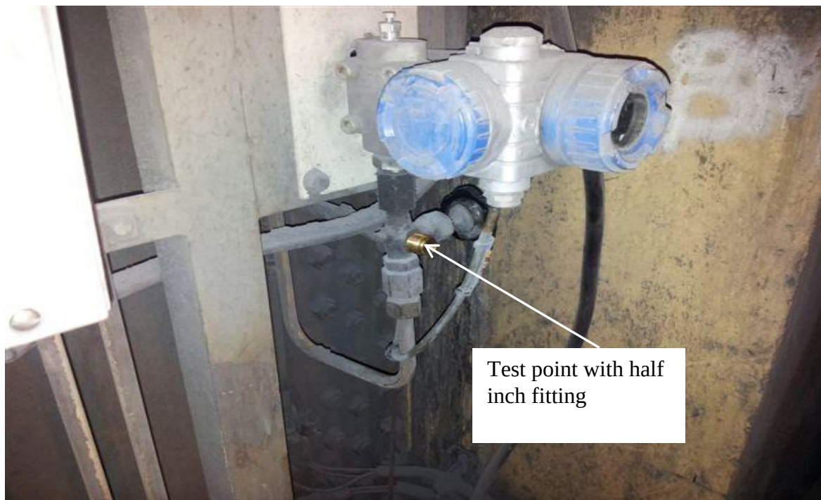
Figure 3-8: Pressure transducer test point at vacuum dried Power Station B
