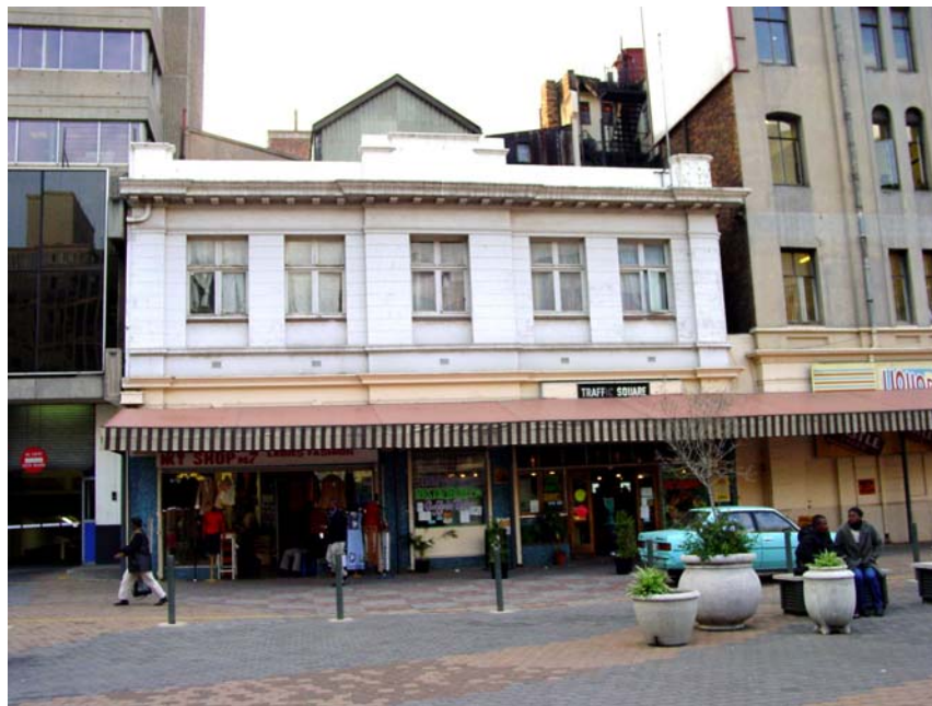
Figure 14: Somerset House, with the Traffic Square Tea Restaurant at street level
