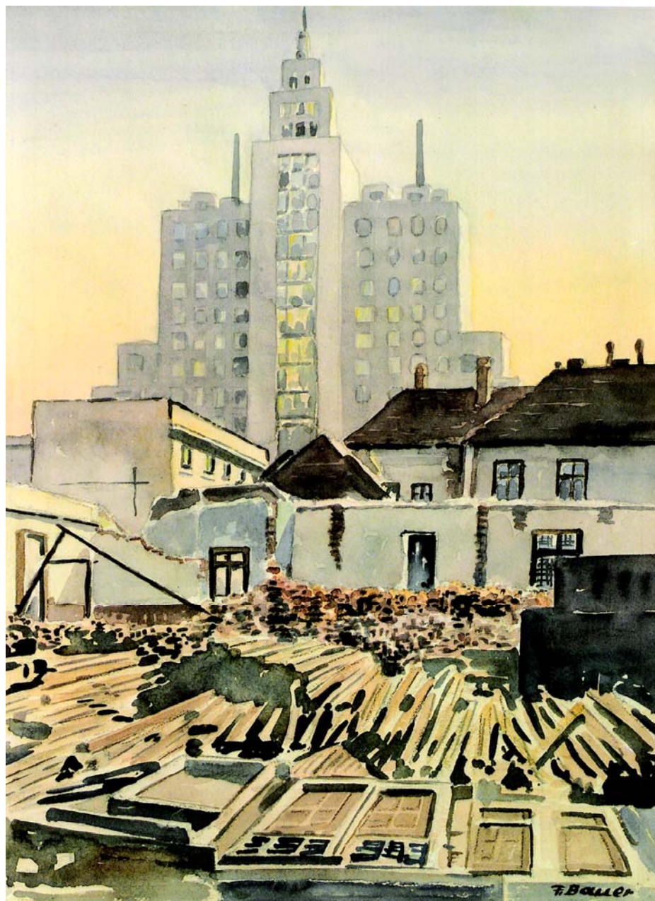
Figure 5: Demolition of the Law Courts, overlooked by Eskom House, 1948.
