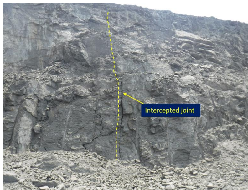
Figure 34: Main face orientation on the northern side: Strike = 297^\circ and Dip = 76^\circ East
