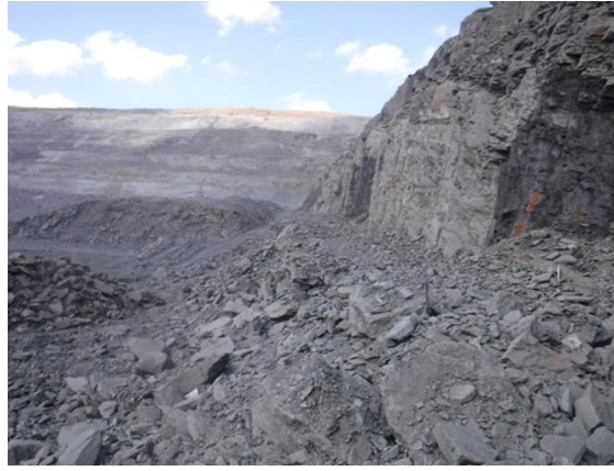
Figure 40: Poor pre-split blast on the 1112 RL
