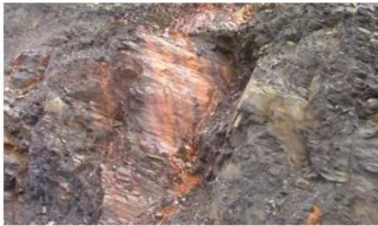
Wedge failure- Effect on geological discontinuity
