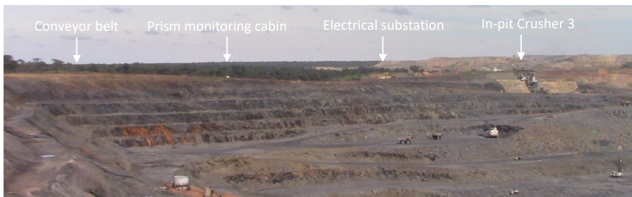
Figure 2: Western final wall and the infrastructure that lies above it
