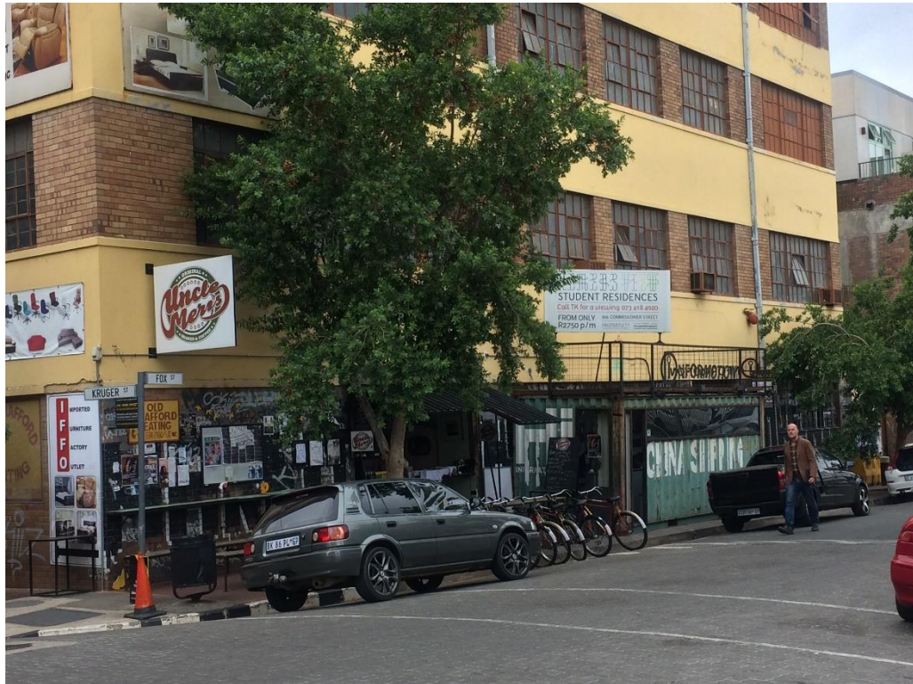
Figure 5.10: Information Centre on Fox street, photograph above depicts pedestrian walking in the street to get past the centre. (Source: Mikhaela Sack. 2015)
