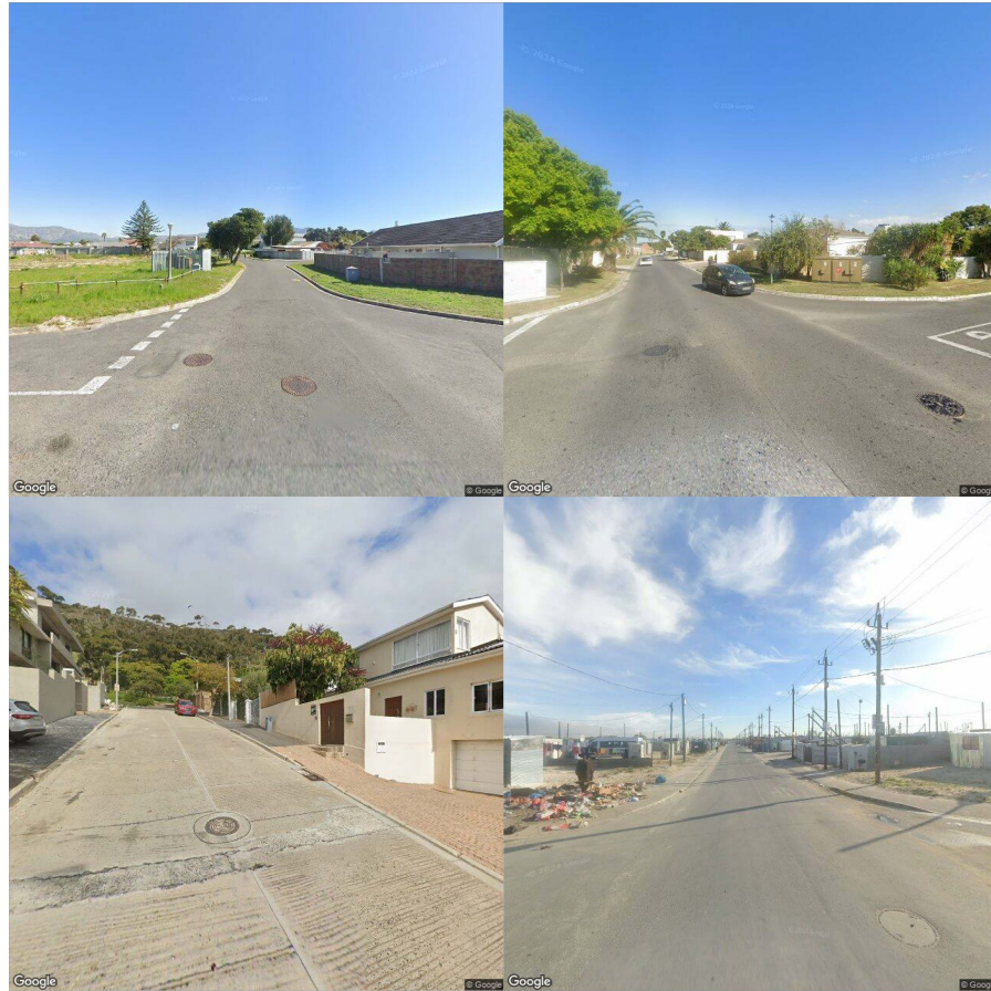
FIGURE 3.19: Manhole covers as a cause for false positives in pothole detection
