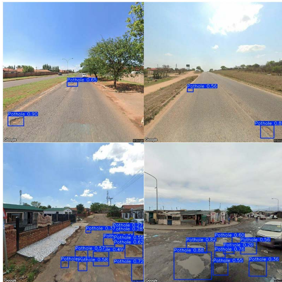
FIGURE 4.2: Images showing variability in confidence scores due to pothole non-conformity and distance from the camera
