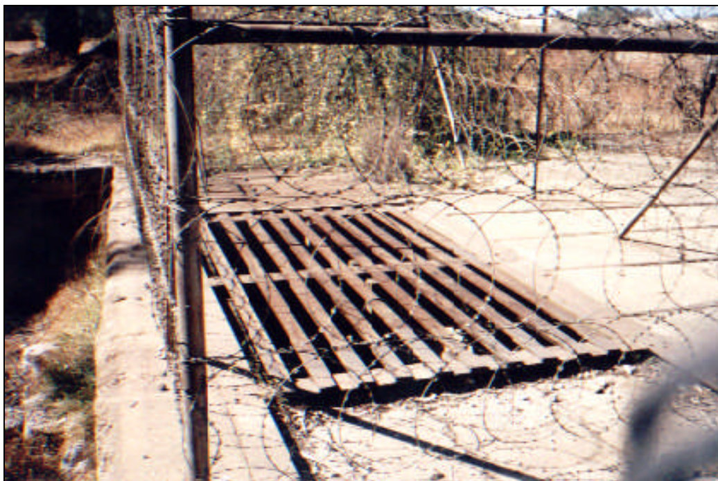
Figure 4.10: Mine opening (S & J 8) sealed with a metal grate and barbed wire fencing, Johannesburg
