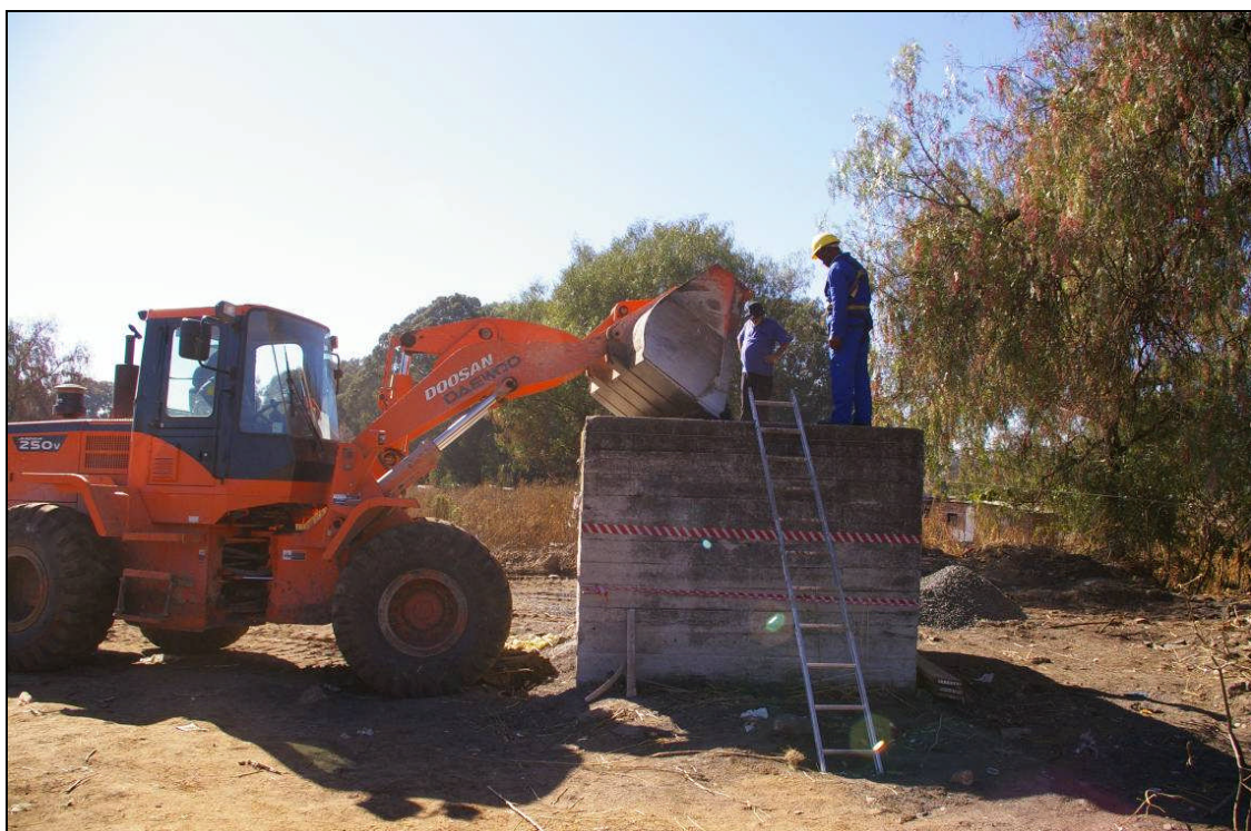
Figure 5.10. S & J 15B: Gravel load being placed on PUF plug
