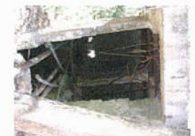
228. South Deep Shaft
