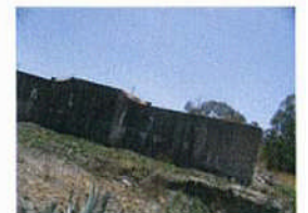
30. Crown Mine 12 Ventilation shaft b
