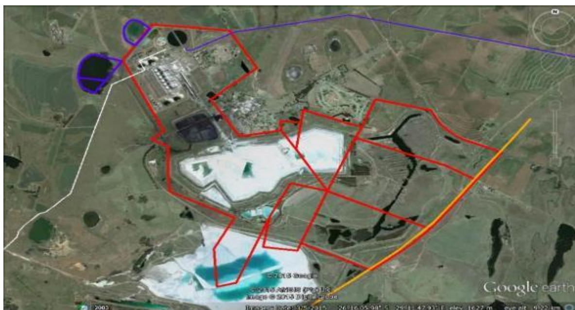
Figure 3.1: Kriel Power Station site boundary (marked with red)
