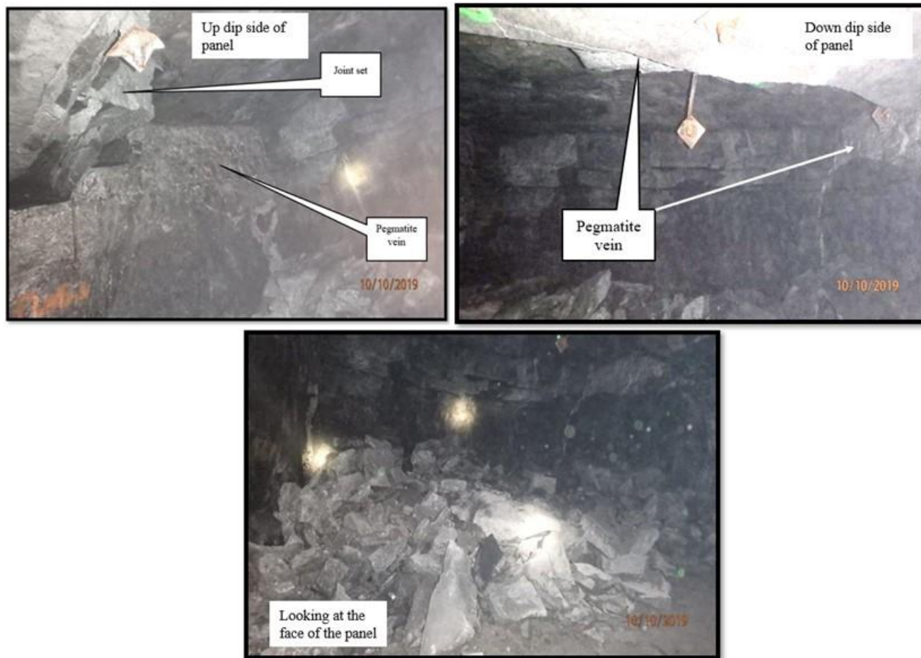
Figure 5-1. Central shaft 10w panel 4 FOG within the face area (Macebele, 2019).
