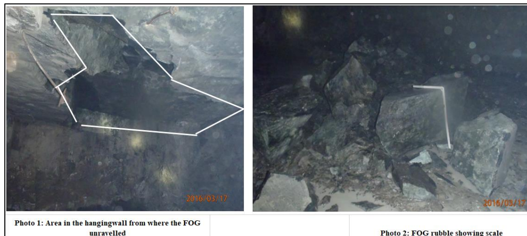
Figure 2-16. Photo of FOG that resulted from chromitite parting, vertical joints and water (Matsobane, 2016b).
