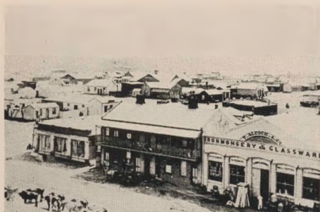
PRITCHARD STREET, 1889, corner of Rissik Street, showing buildings on the present Stoffords' site. The tower of St. Mary's Hall is in the middle distance. "A hive of industry and a nursery of great expectations."
