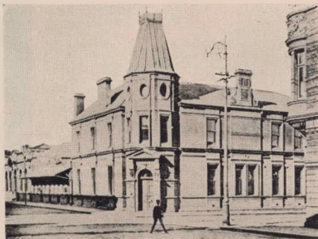
THE BANK OF AFRICA, the first building on the corner of Commissioner and Harrison Streets.
