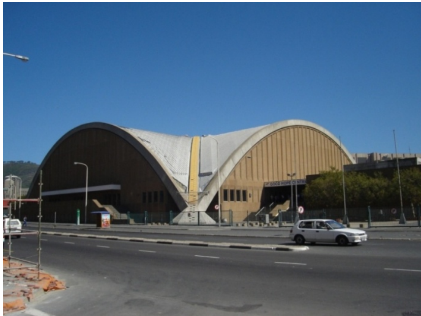
Figure 1.1 - Cross vault structure (Good Hope Centre, Cape Town)
