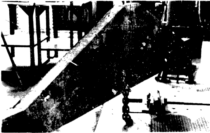
Figure 4.2(a) View of 800mm deep variable section beam being manoeuvred onto test bed (series F2)
