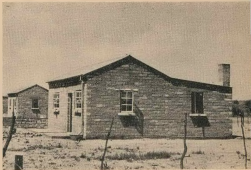
Municipal houses at Warmbaths Location constructed of breeze concrete blocks.
