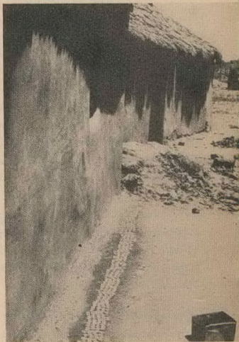
A paving of crown corks to take drips from a thatched roof.
