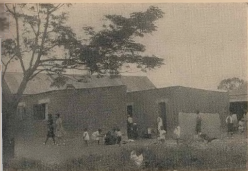
The incorporation of lodgers rooms has caused overcrowding in Pietersburg Location, where, however, the houses are well built.
