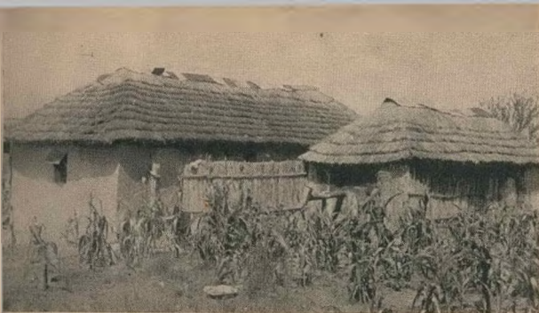
The mud plastered house with thatched roof. In this example the kitchen is in the separate building. Note the canopy over the unglazed window.
