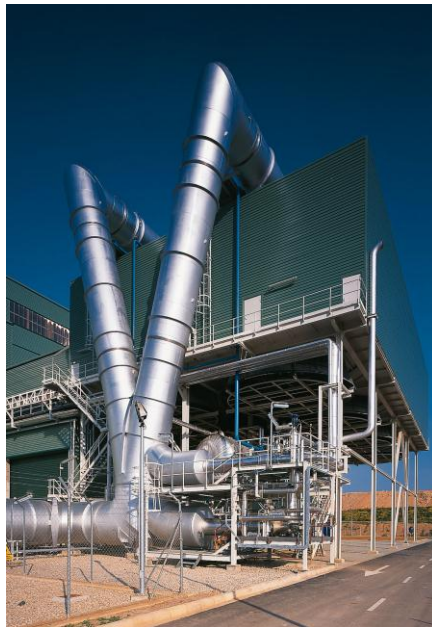
Figure 1.6: A direct dry-cooling system
