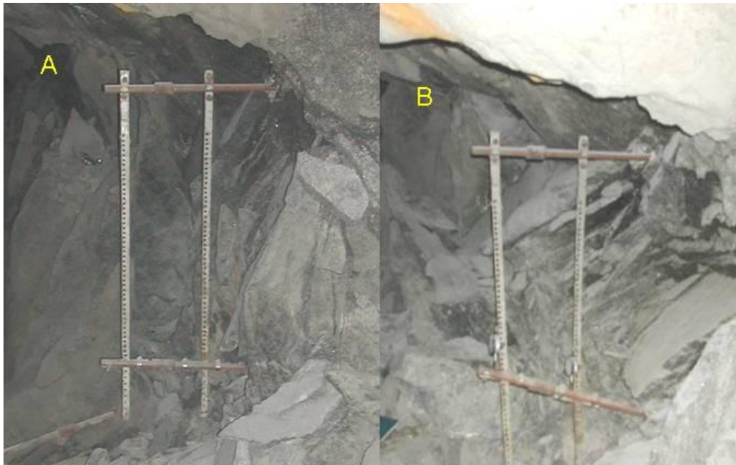
Figure 4-60 Amandelbult site: rotation of jumpers grouted into the centre of P2 near the top edge of the pillar and about 1 m vertically below. A = pillar failure; B = three months after pillar failure
