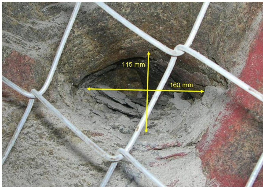
Figure 4-71 Impala site: blasthole sockets indicating a k-ratio of about 1.4
