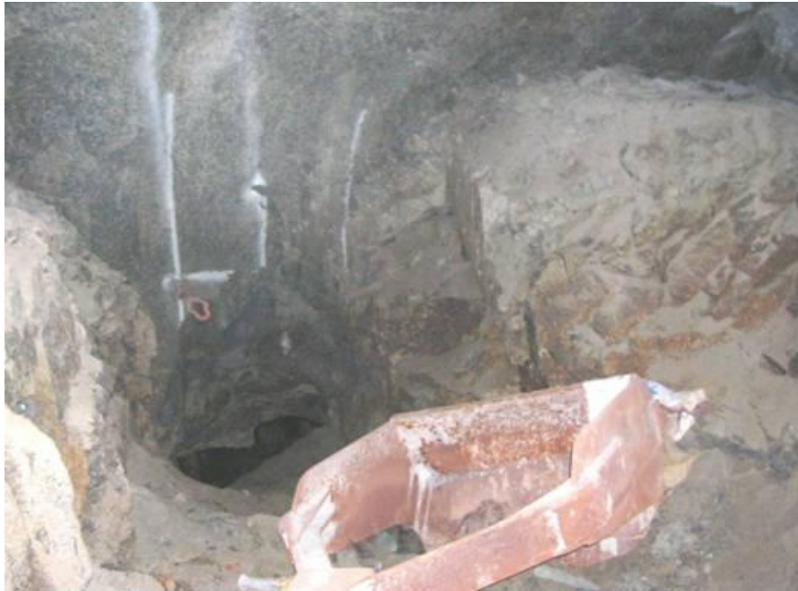
Figure 4-74 Impala site: holing slot cut through the siding from the ASG, after pillar failure. P1 is to the right of the photograph
