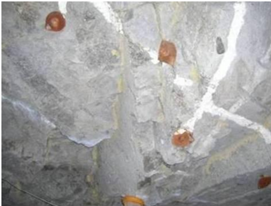
Figure 2-12 Union site: blocky hangingwall adjacent to the isolated pillar
