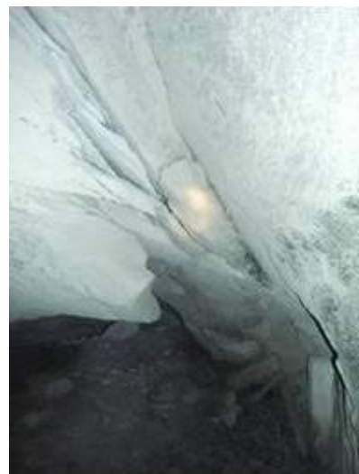
Figure 4-5 Gothic arching and extension fracturing observed in the hangingwall of an in-panel raise
