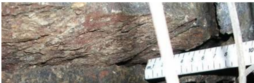
Figure 4-69 Impala site: strata-parallel fault observed in the travelling way, about 1.3 m below the stope
