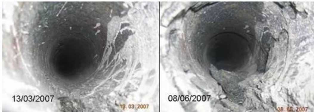
Figure 5-110 Deterioration of the inspection borehole in Union P1 before mining initiated (left) and just before pillar failure (right)
