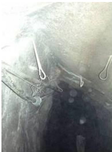
Figure 4-5 Gothic arching and extension fracturing observed in the hangingwall of an in-panel raise
