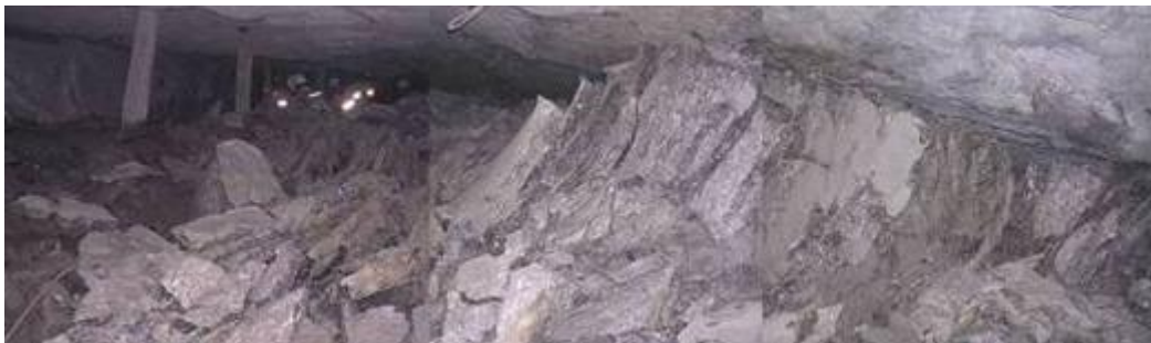
Figure 5-129 Panoramic view showing the up-dip end of a burst pillar. Note the gully is full of rock fragments from the pillar burst
