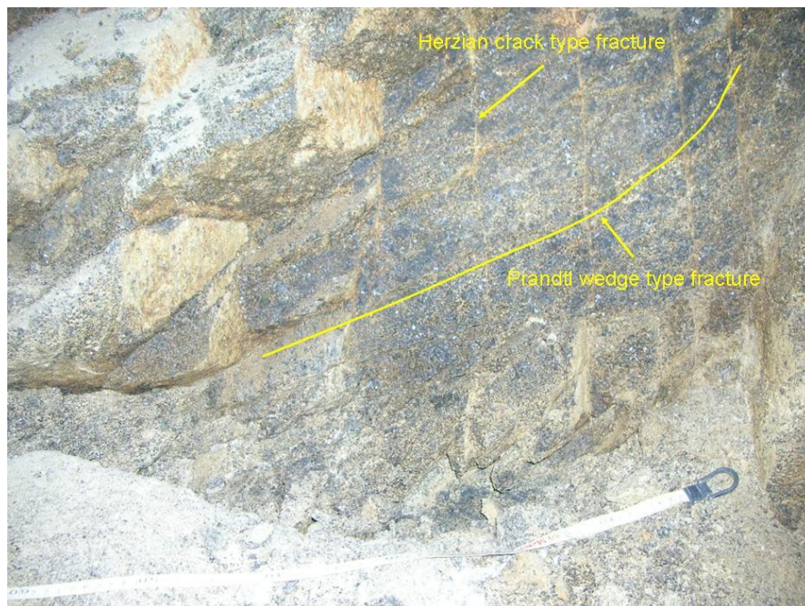
Figure 4-75 Impala site: fracturing and jointing observed in the slot adjacent to P1. The fracturing was exposed when a holing was cut through the footwall after pillar failure. The yellow line indicates the position of a shallow-dipping, curved fracture. Vertical fractures can also be seen
