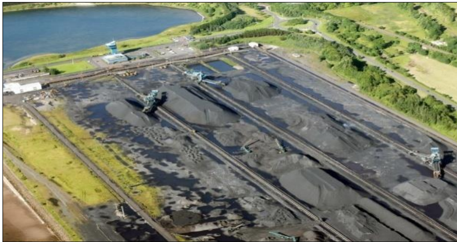
Figure 2-23: Coal stockyard with poor drainage (Hunterson, 2013)
