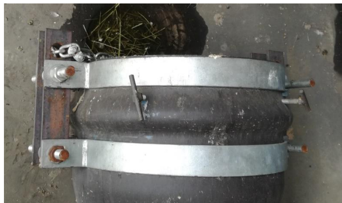
Figure 3-6: Drainage pipe suspension bracket
