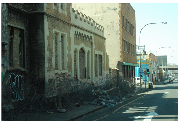
Figure23: Abandoned buildings allegedly occupied by homeless people (Conco,2015)
