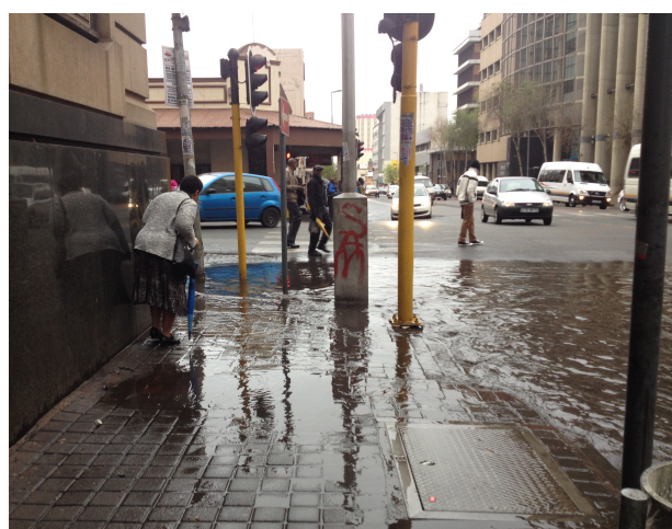
Figure25: Poor drainage (Conco,2015)
