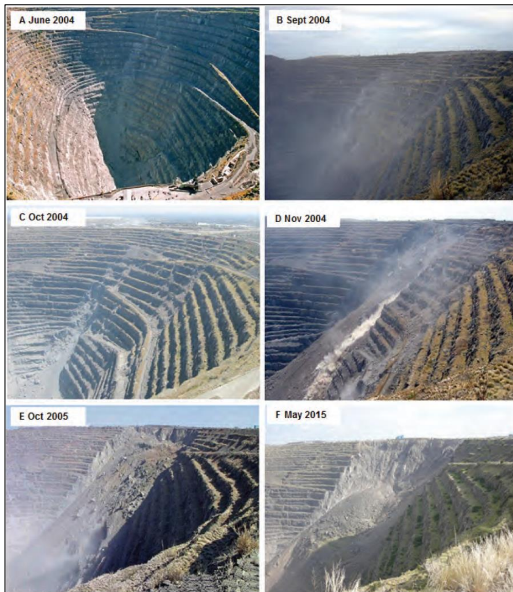
Figure 26: Evolution of the north wall failure (north-west view)
