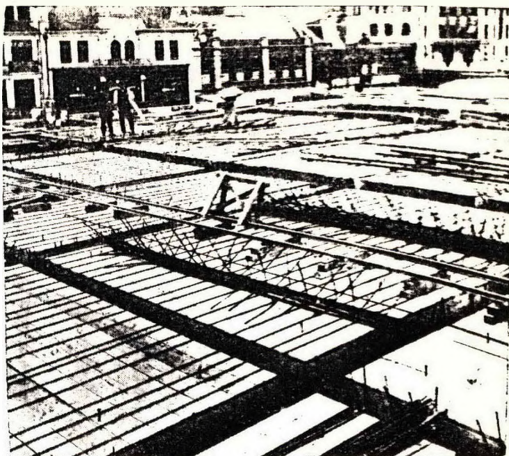
Reinforced Concrete Beams, Slabs and Columns on "KAHN" System, Town Hall, Johannesburg
