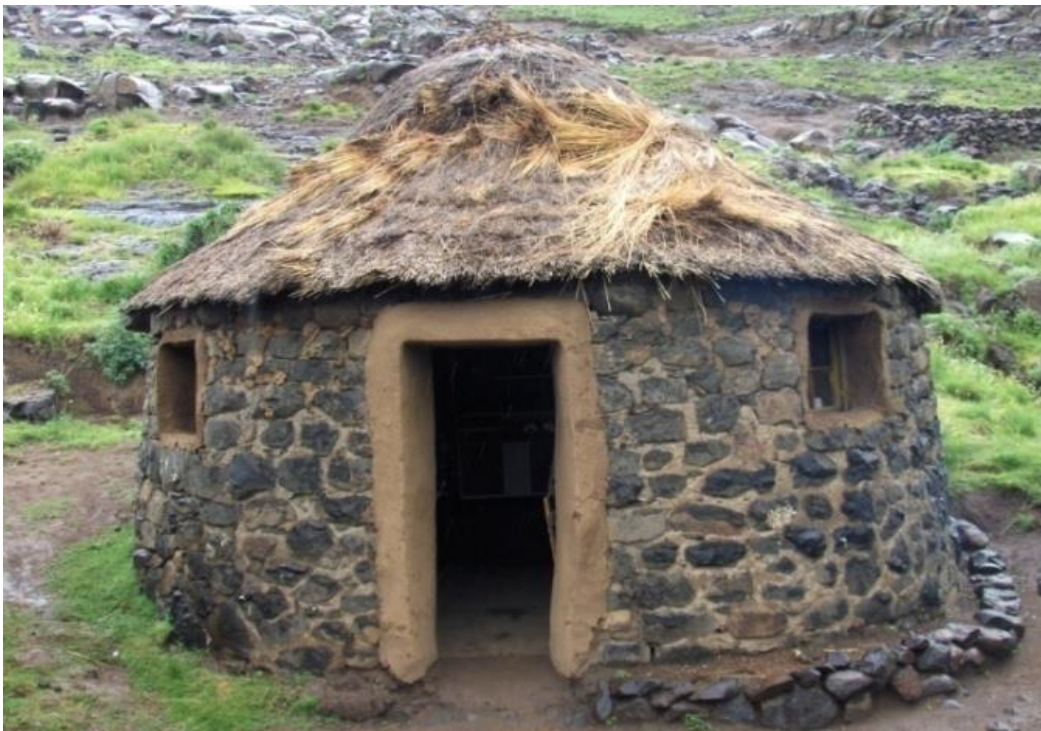
Figure 5.42: Grass thatched Mokhorro house (January, 2010). Source: Own photo
