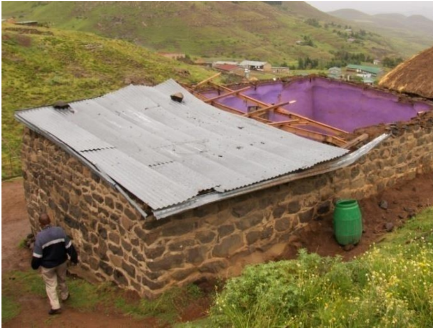
Figure 5.41: Wind prone roofing in Phamong, Mohale's Hoek (January, 2010). Source: Own photo.
