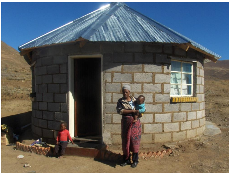
Figure 5.46: Wind resistant house built from sturdy materials in Moyeni, Quthing (July, 2010).
