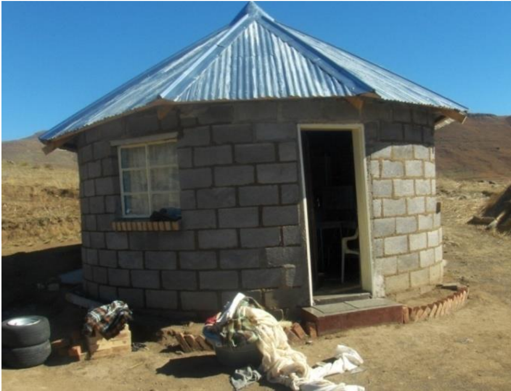
Figure 5.43: Newly built houses with wind resistant pitched roofs in Mphaki-Quthing (July 2010).
