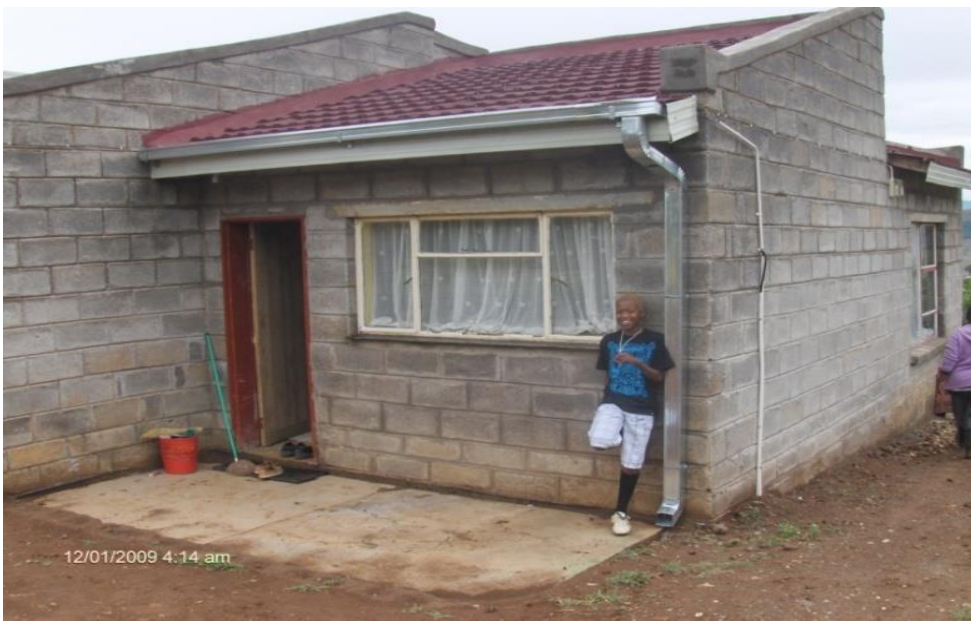
Figure 5.44: Recently built house with Harvey tiles and wind resistant roofing in Moyeni, Quthing (February 2010).
