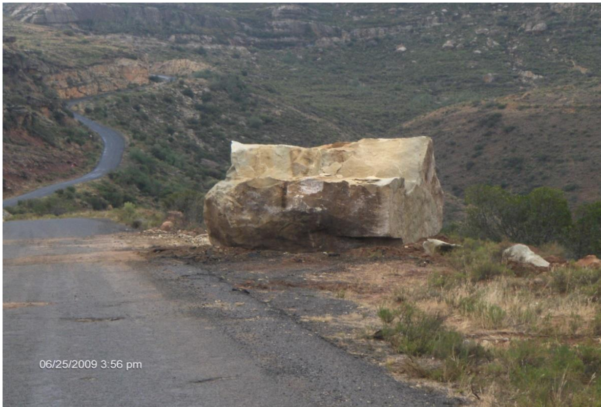
Figure 5.14: Rock falls caused by excess rainfall at Mphaki Quthing. (25/06/2009) Source: Own photo
