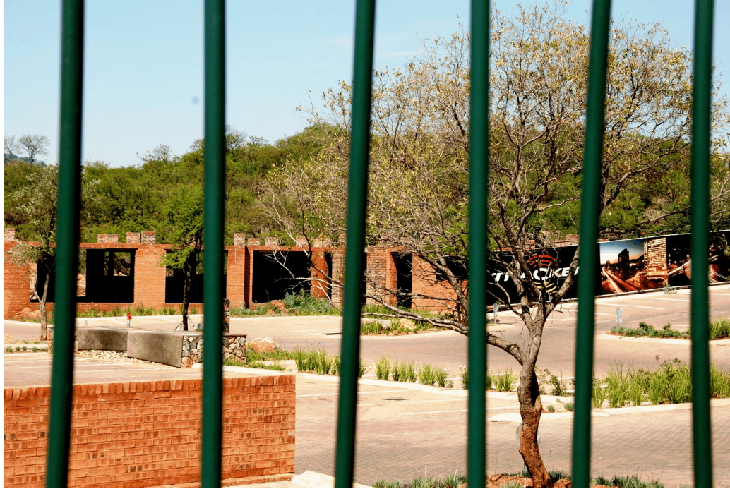
Figure 5. Darrenwood site, now just a koppie surrounded by an office park.
