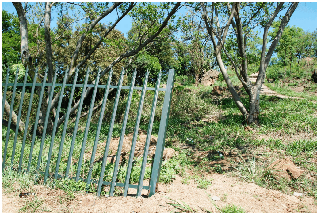
Figure 2. Emma Park was considered as part of the Darrenwood area. An attempt has been made to fence off this urban park, but, as can be seen, the fence was damaged but has subsequently been repaired.
