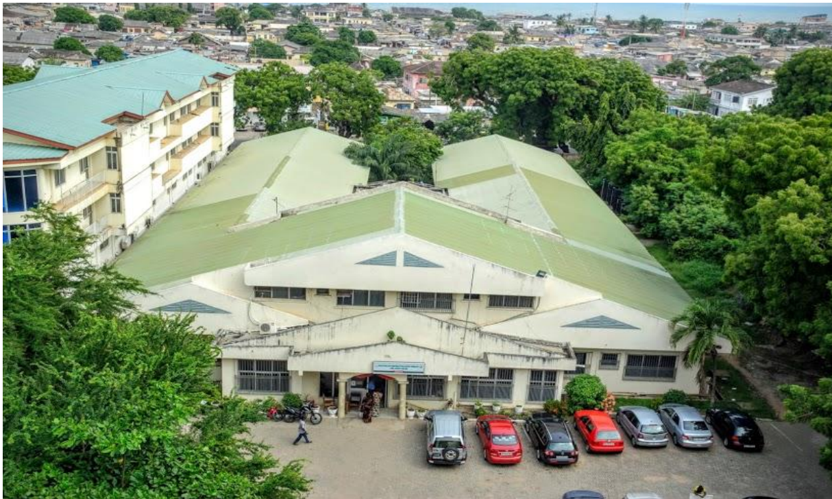
Figure 3.2: The building of the NRPS & BC of KBTH
