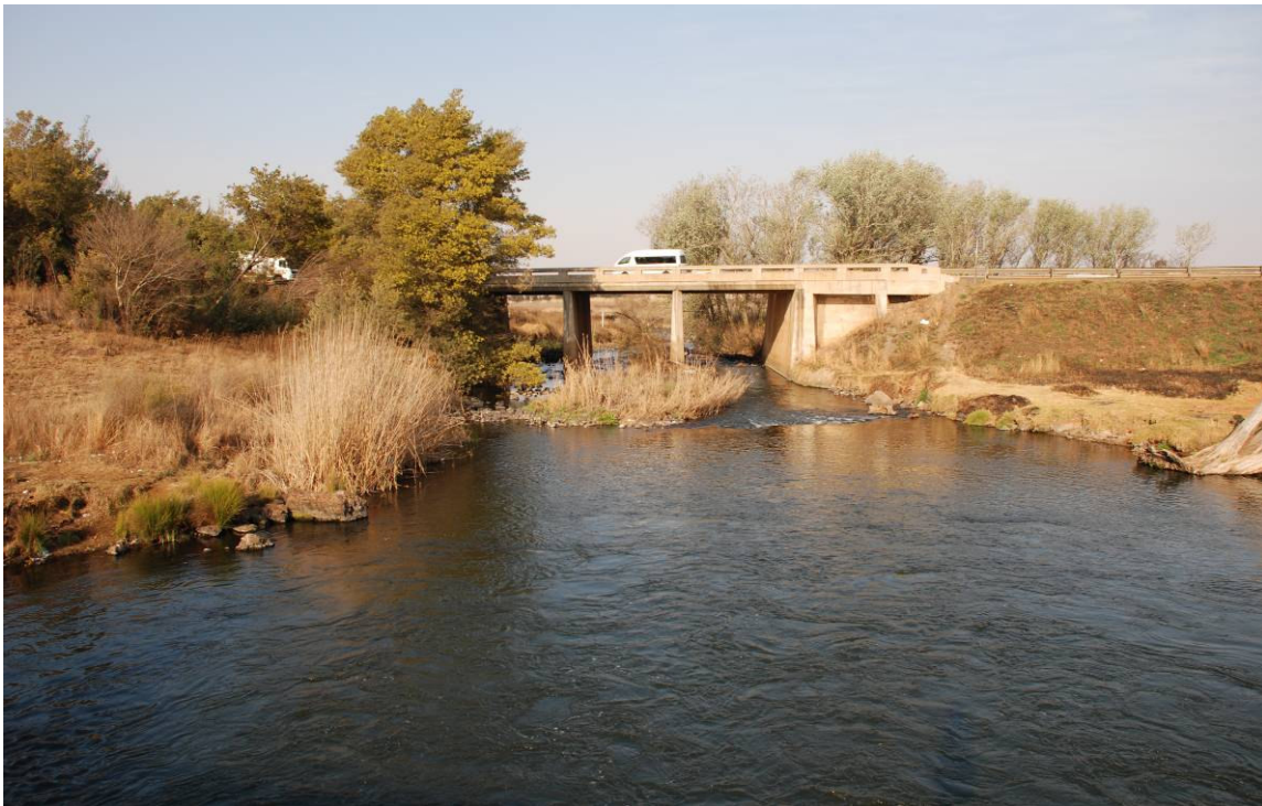
Figure 5.1.9: Point A: Channel cut after the Olifantvlei discharge point (Golden Highway in background; August 2008).
