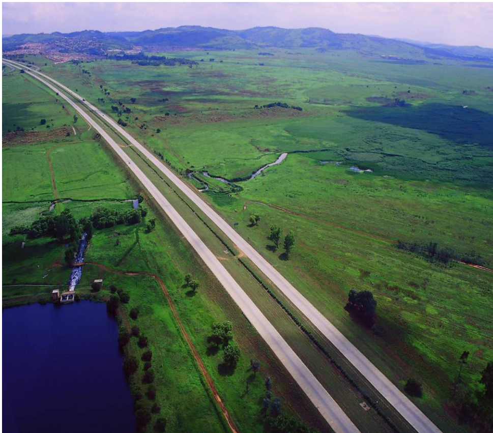
Figure 3.4.2: Discharge point of the Bushkoppies sewage treatment plant ponds into the Klip River Wetland (courtesy of T.S. McCarthy, November 2007).
