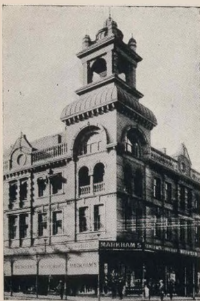
LEFT: Markham's branch in Corporation Buildings, corner of Rissik and Commissioner Streets. RIGHT: RISSIK STREET. 1889. An early print showing Palace Buildings, a well-known landmark today, designed by Mr. J. S. Donaldson. Rissik Street was an important shopping area, especially in the 'nineties.
