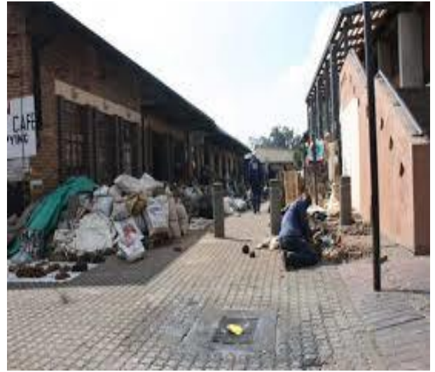
Picture 3: Wolhuter Hostel next to hostel to informal settlement (Source own photos)
