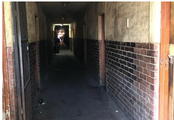
Picture 17: passage / hallway of a single block
