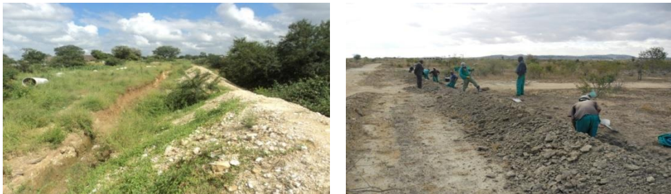
Photos above shows: left, a trunk sewer line under construction and right, a major waterline to project site.
